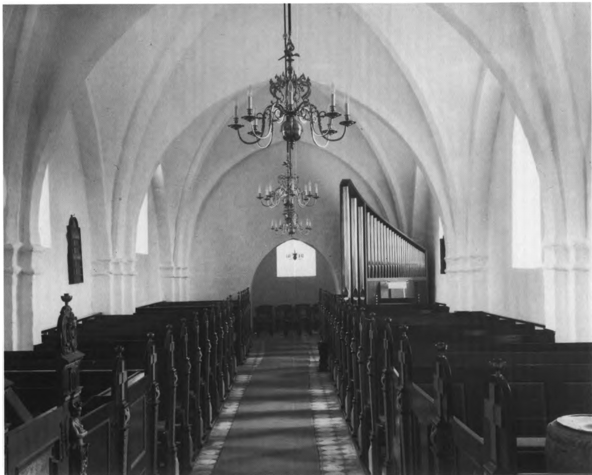
Fig. 6. Indre, set mod vest. NE fot. 1981. - Interior to the west.
